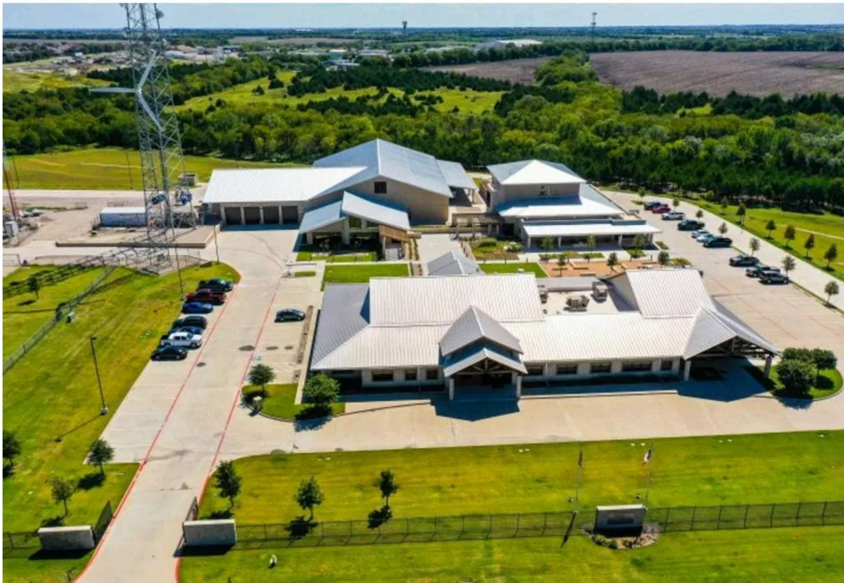
Rayburn Electric Cooperative's headquarters in Rockwall, Texas. RAYBURN ELECTRIC COOPERATIVE
